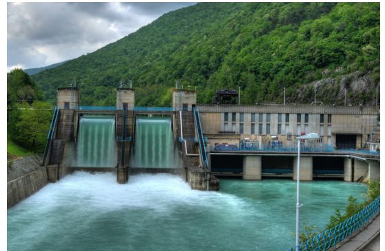
Figure 1. Hydroelectric Power Station
